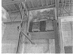
Some distribution panels and receptacles in the medicinal marihuana production area are missing cover plates, exposing live electrical wires.
