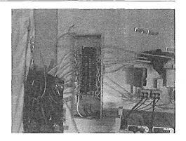
Loose live wiring, unsecured junction boxes and receptacles and missing lighting fixtures were overserved throughout the Green Island Trading Company tenant spaces.
