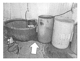
.3 It appears that water is sprayed directly onto the plants and floor slab using a garden hose. Water may penetrate the concrete slab and cause corrosion of the underlying steel deck and supporting structure.
