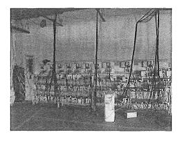
The electrical power supply to the medicinal marihuana production area uses temporary wiring.
