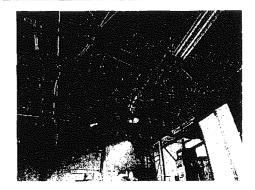
.2 In isolated locations, fireproofing material at the underside of the second floor framing is damaged/missing. Damaged fireproofing requires immediate repair.
