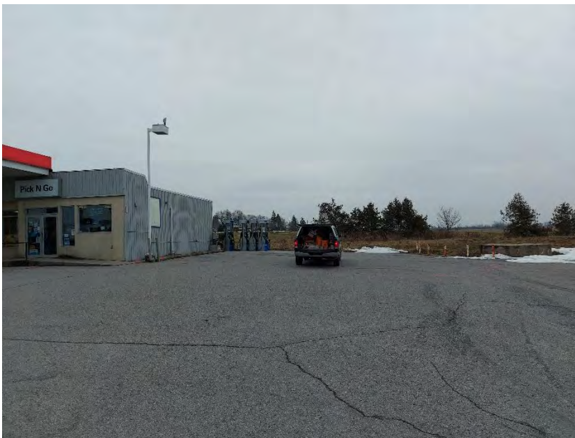
Looking south towards the west portion of the site
