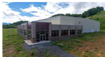
Polycap LLC will establish its first U.S. manufacturing facility in the 76,000-square-foot Russell County shell building in Lebanon, VA. (Photo: Russell County Industrial Development Authority)
