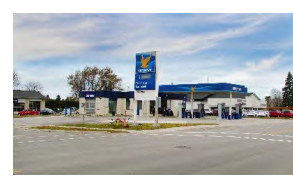
SOLD & CLOSED $1,300,000 274 Bayfield Road, Goderich Vendor: Superior Court of Justice Vacant former Ultramar gas station and automated car wash facility.
