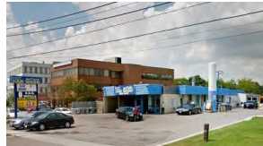
SOLD & CLOSED $3,700,000 5462 Dundas Street West, Toronto Vendor: Superior Court of Justice Single storey car wash facility.
