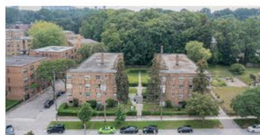
290-292 The Kingsway 44 units
