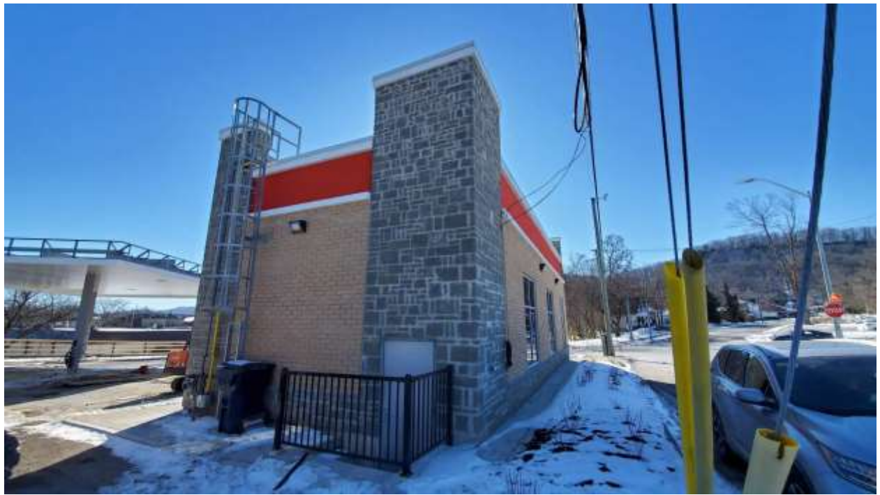
Northwest Elevation of Subject Building
