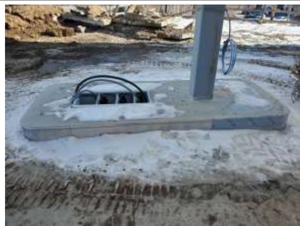
Fuel Dispenser Pad
