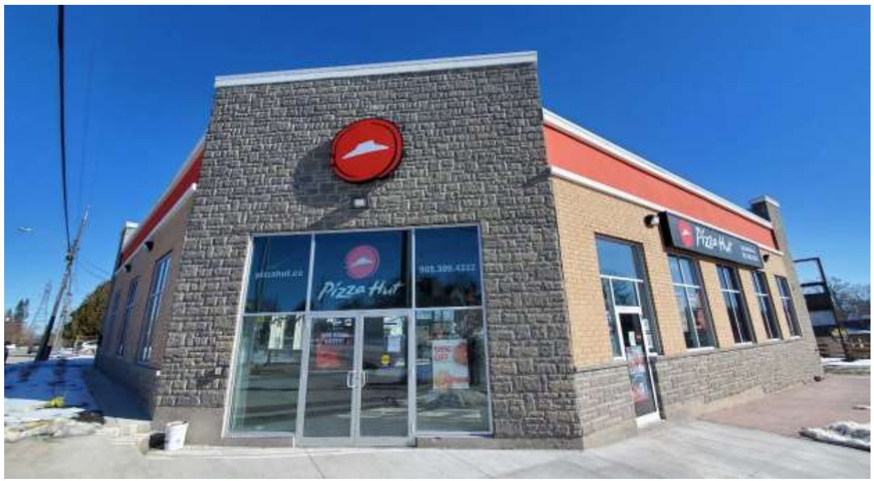
Southwest Elevation of Subject Building
