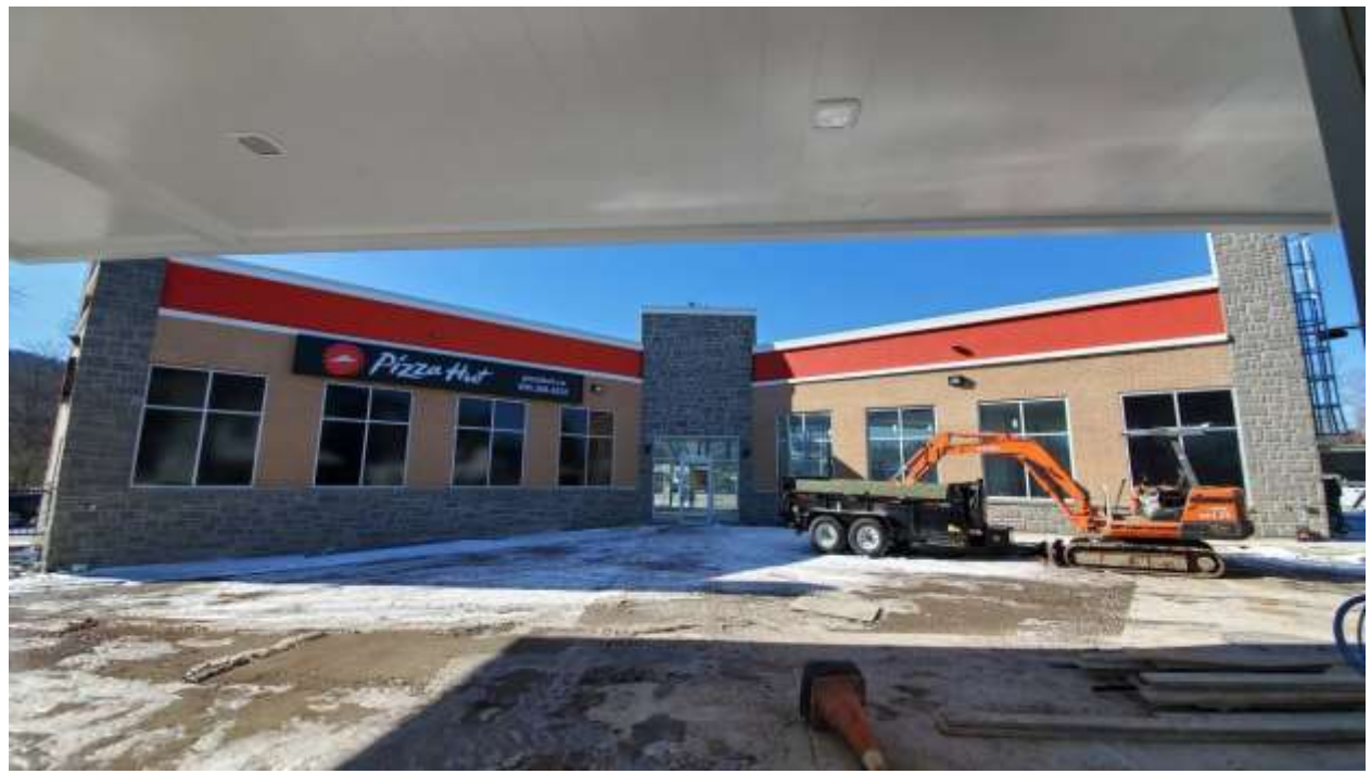
Front (East) Elevation of Subject Building
