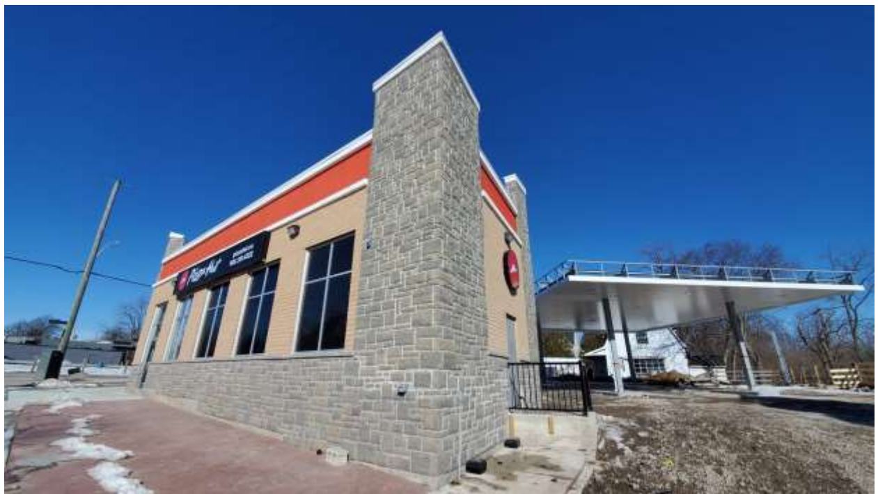
Southeast Elevation of Subject Building
