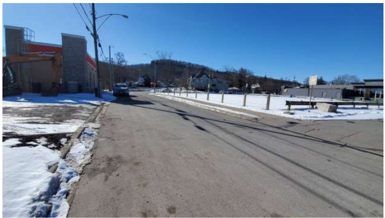
South View of Patton Street
