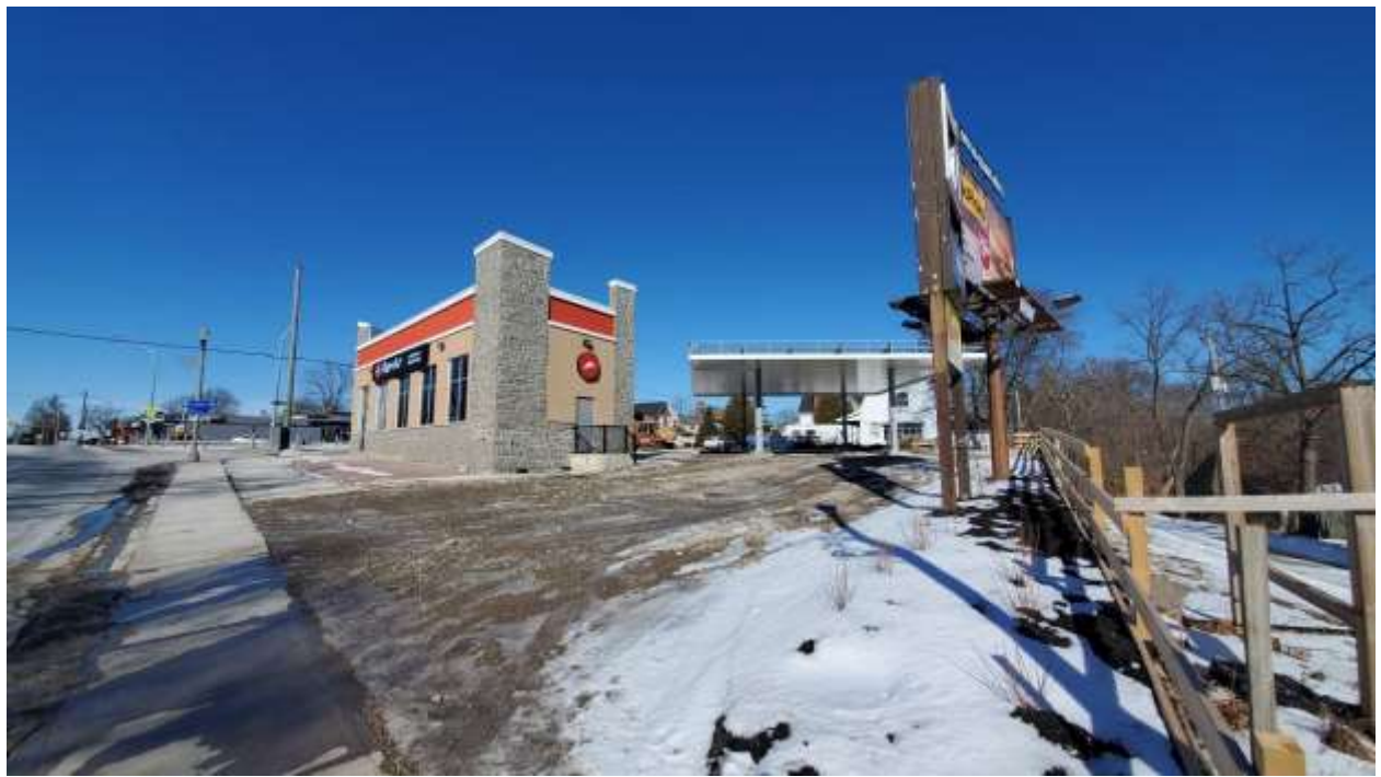
Southeast View of Subject Property
