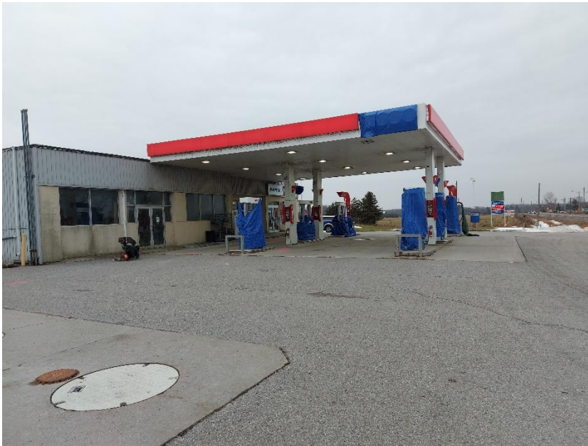
Looking southwest towards the east portion of the site
