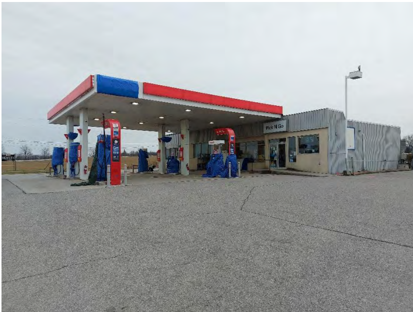
Looking southeast towards the west portion of the site
